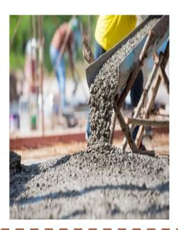
Concrete is a construction material composed of cement, fine aggregates (sand) and coarse aggregates mixed with water which hardens with time. Portland cement is the commonly used type of cement for production of concrete. Concrete technology deals with study of properties of concrete and its practical applications.
