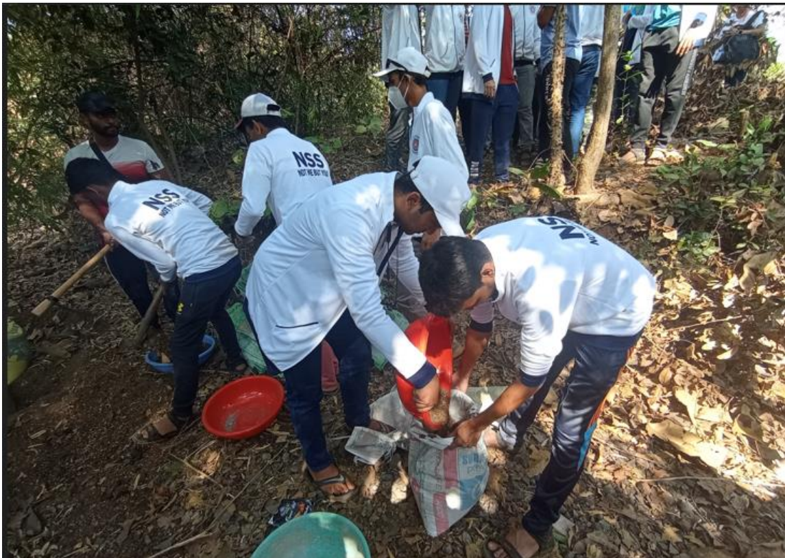
Bund Dam Construction Activity 2022-23
