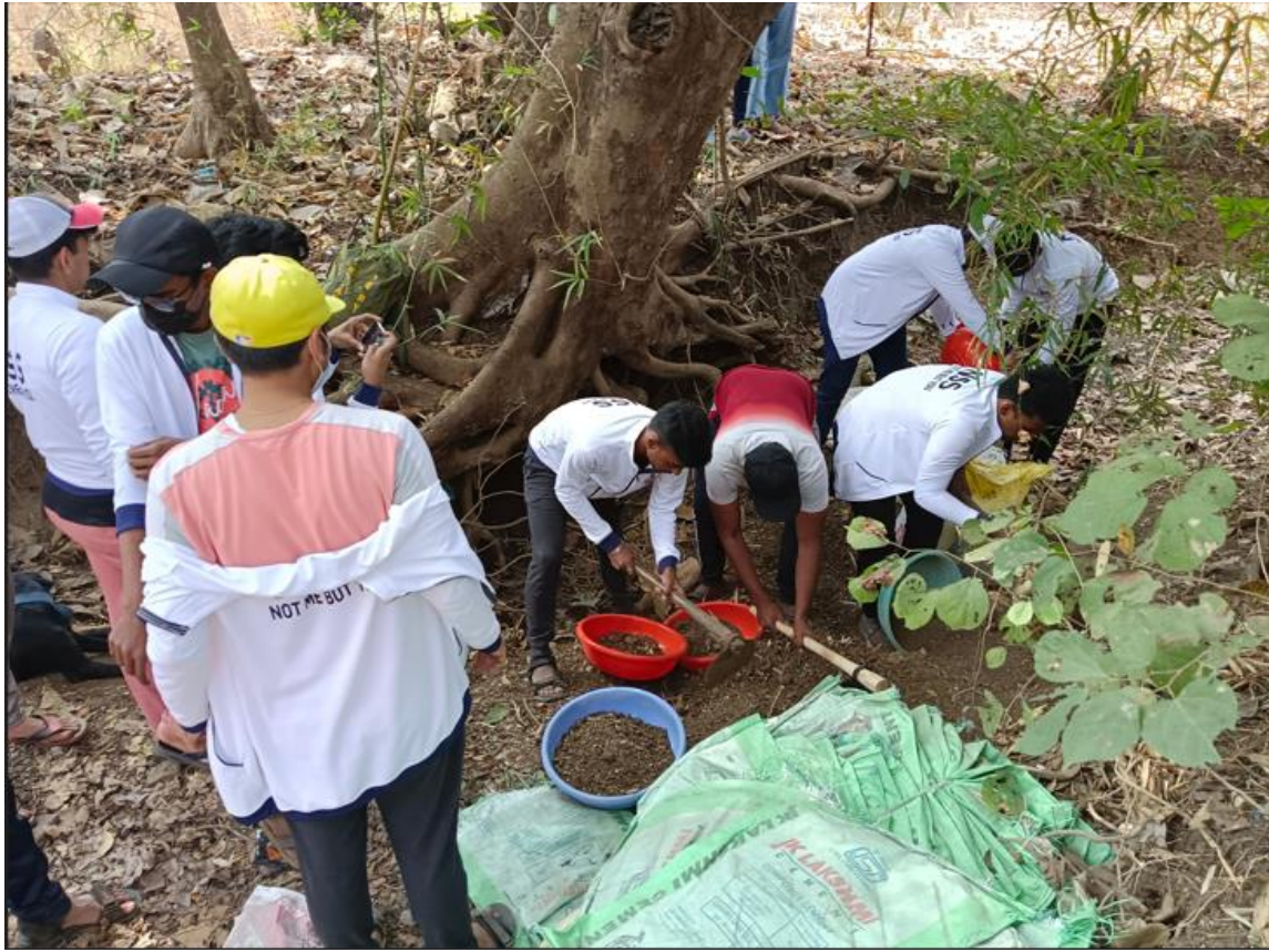
Bund Dam Construction Activity 2022-23
