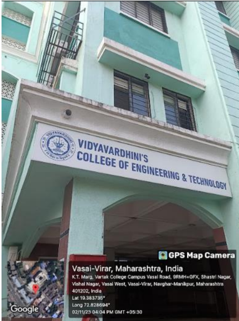
CCTV Camera (Capture Gate View)
