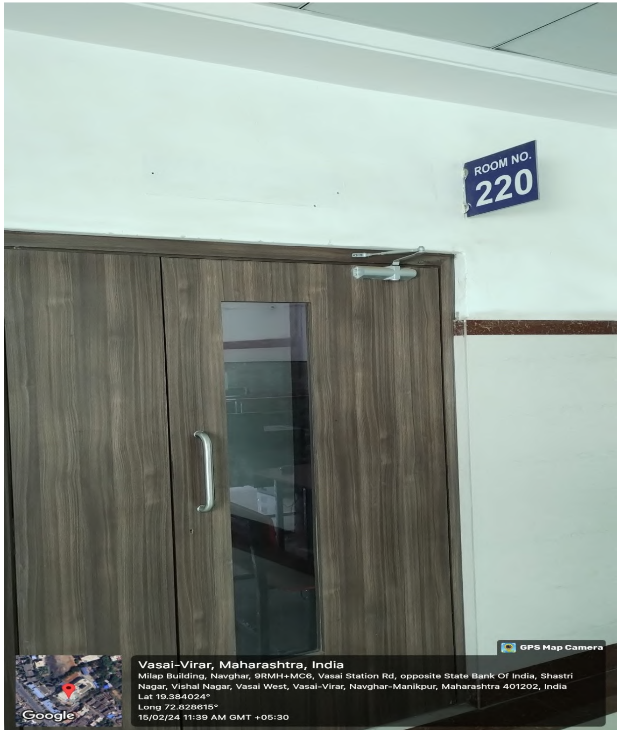
Classroom 220 Outside View
