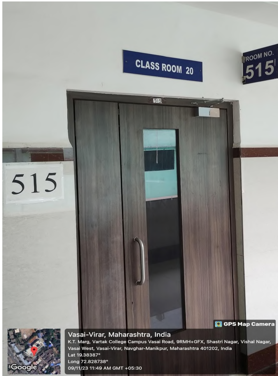
Classroom 515 Outside View
